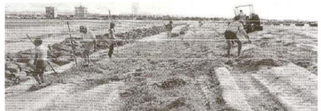
Hand spreading of mulch on Wave Break Island (Source: GCCC 1986)
